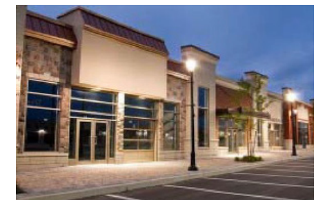
Maintain well-illuminated building frontage and pedestrian pathway.
