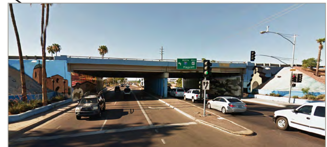
Potential gateway treatments (murals): S. 16th St., at the I-17 overpass, looking south.
