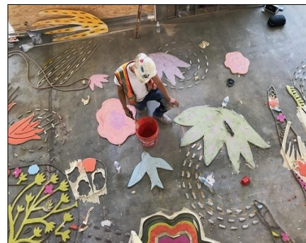
Terrazzo floor specialists pour colorful aggregate mix into the aluminum forms.
