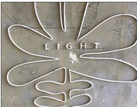
Aluminum strips attached to the floor define the design's various shapes
