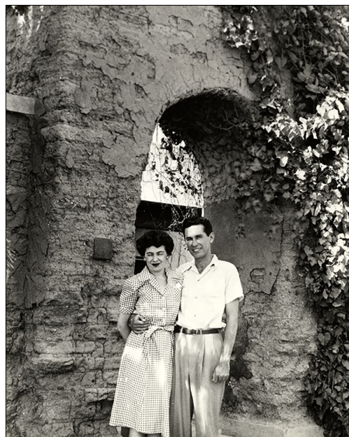
An unidentified couple embrace in front of the chapel. The chapel's exterior stucco has eroded to reveal the handmade adobe bricks beneath, 1940s.
