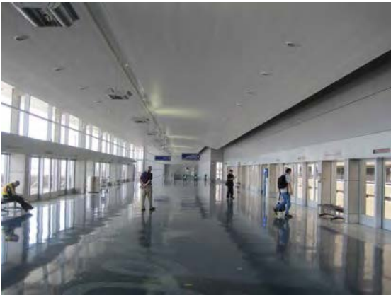
Metal Ceiling Panels at Sky Train
