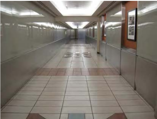
Effective wall areas at International Arrivals. 4' textured stainless steel wainscot with durable finish above.
