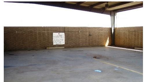
Photo 7-1: PHX Wash Rack
