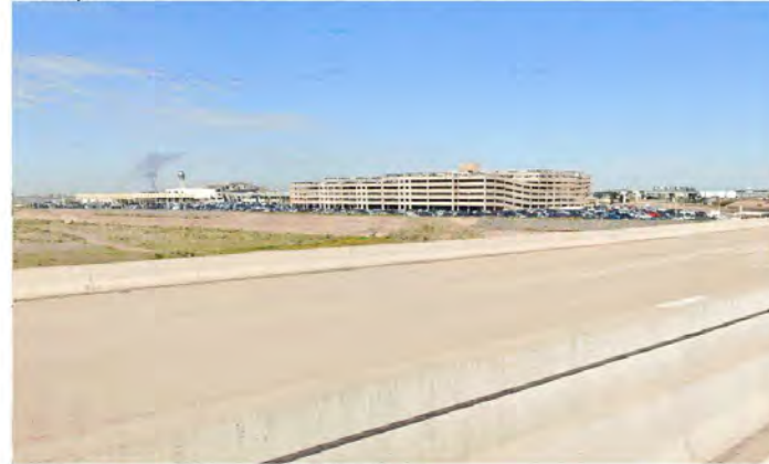
View #5: S. 44th Street bridge over the Salt River looking west towards the Airport
