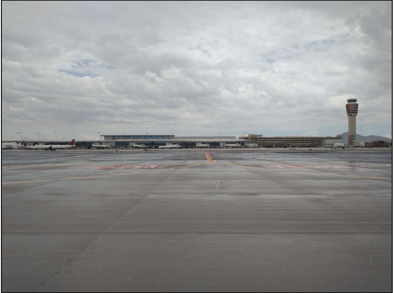
Figure 4. Taxiway 8 location; view facing north.
